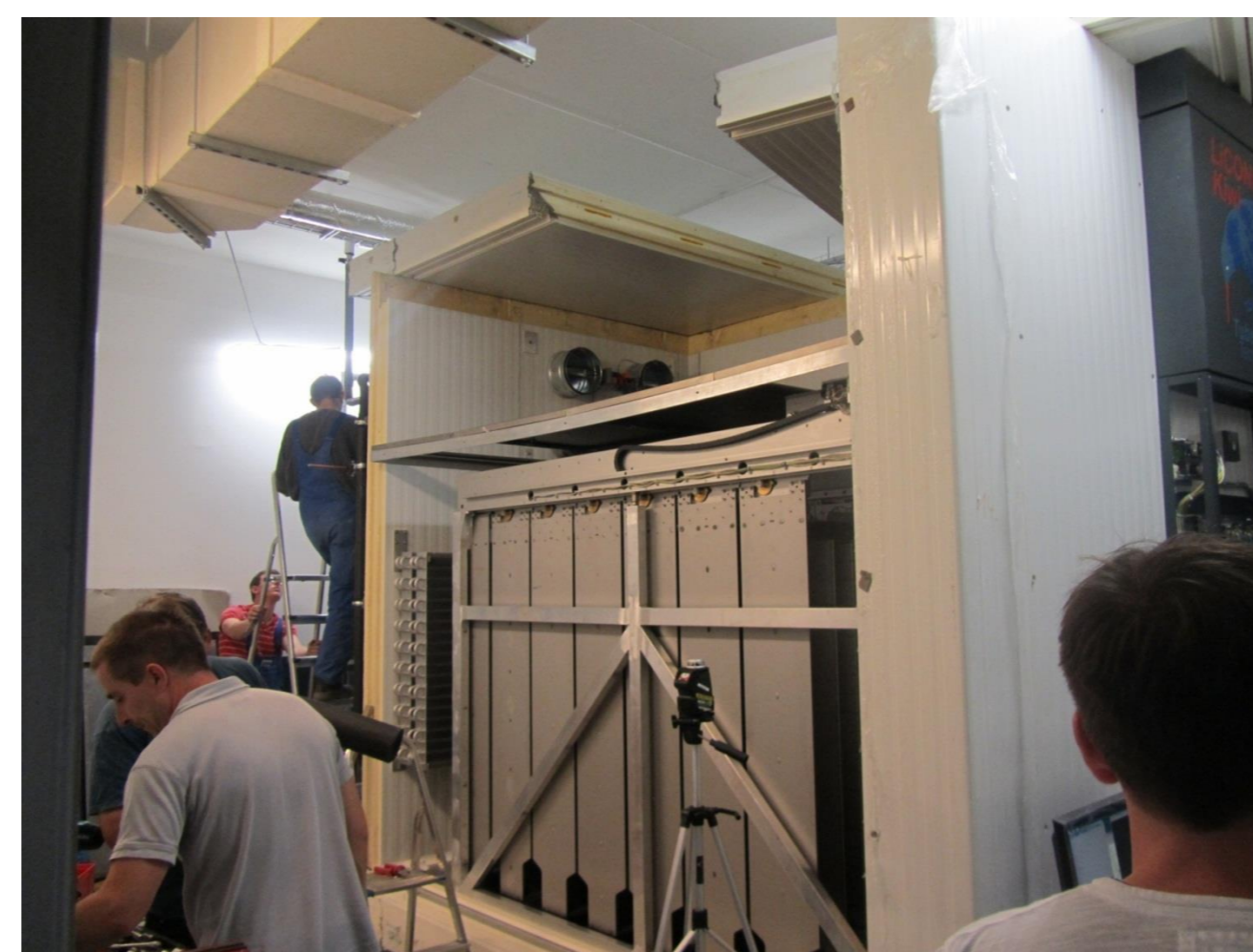
Fig 2. Installation of the 1 st biorepository in Greifswald
